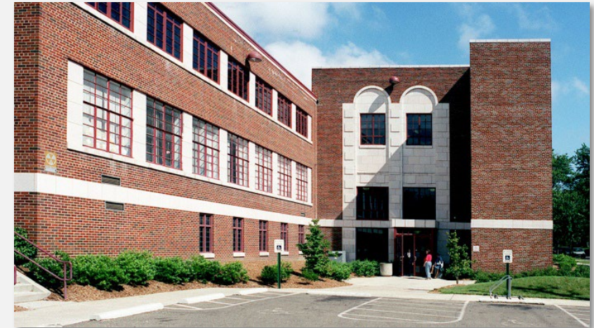
Balch Street Community Center
