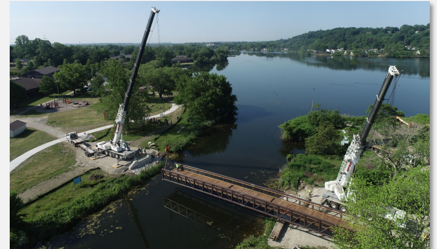
Drone photo of the bridge setting at Summit Lake.
