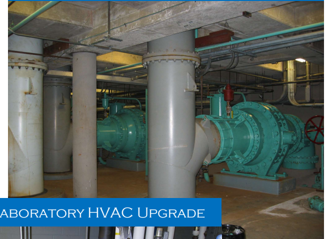
HIGH SERVICE PUMP BALL VALVES
