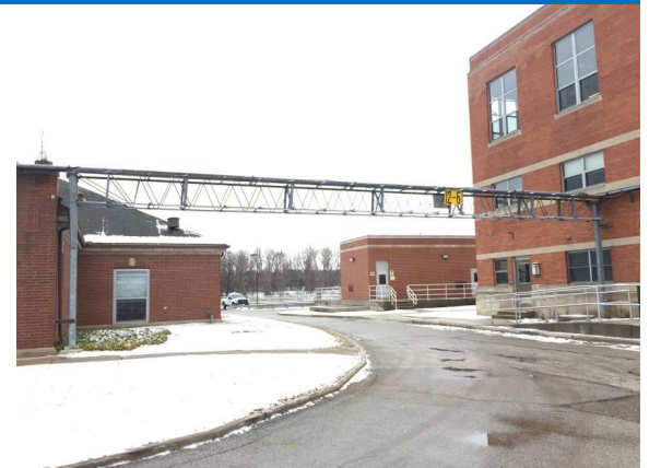
LOW LIFT 5KV FEEDER
