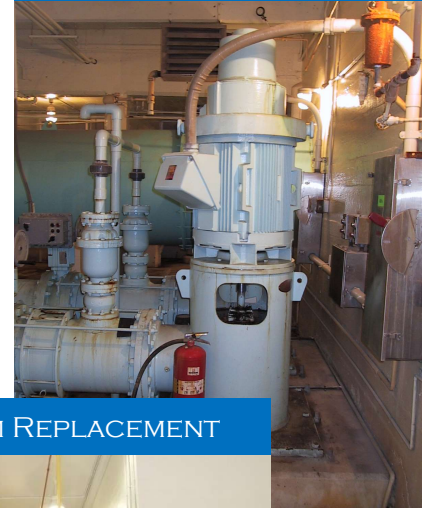
BACKWASH PUMP REBUILD
